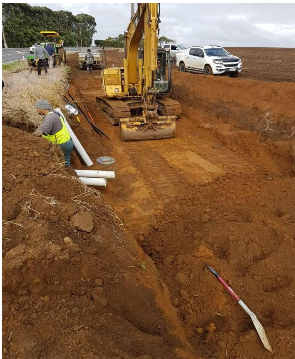
Figure 5. Construction of an SRP following the E&S Control Plan.
