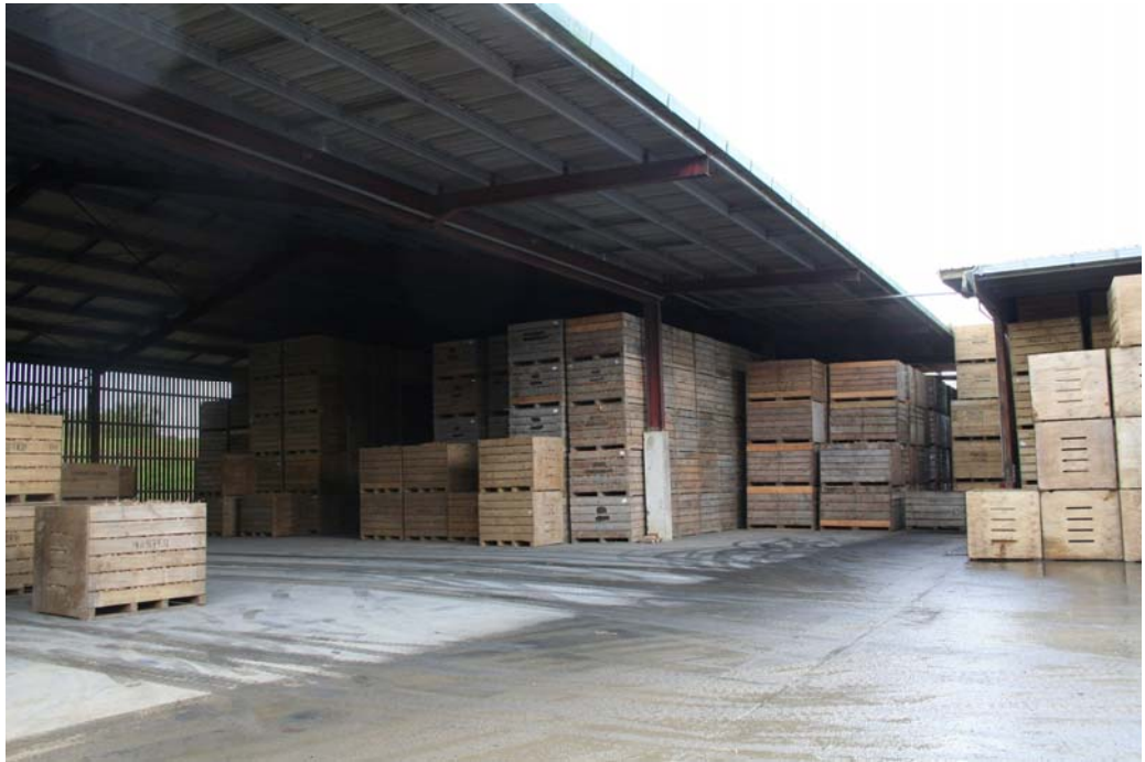
Onion store (showing about two-thirds of one of the two such structures) at Master and Sons.
